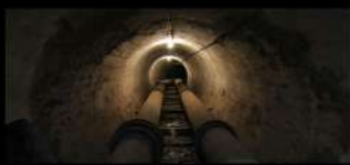
Utility Tunnel Mapping
