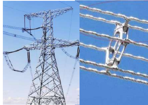
Through AI capabilities, drones can accurately locate defects in power armour clamp during inspections
